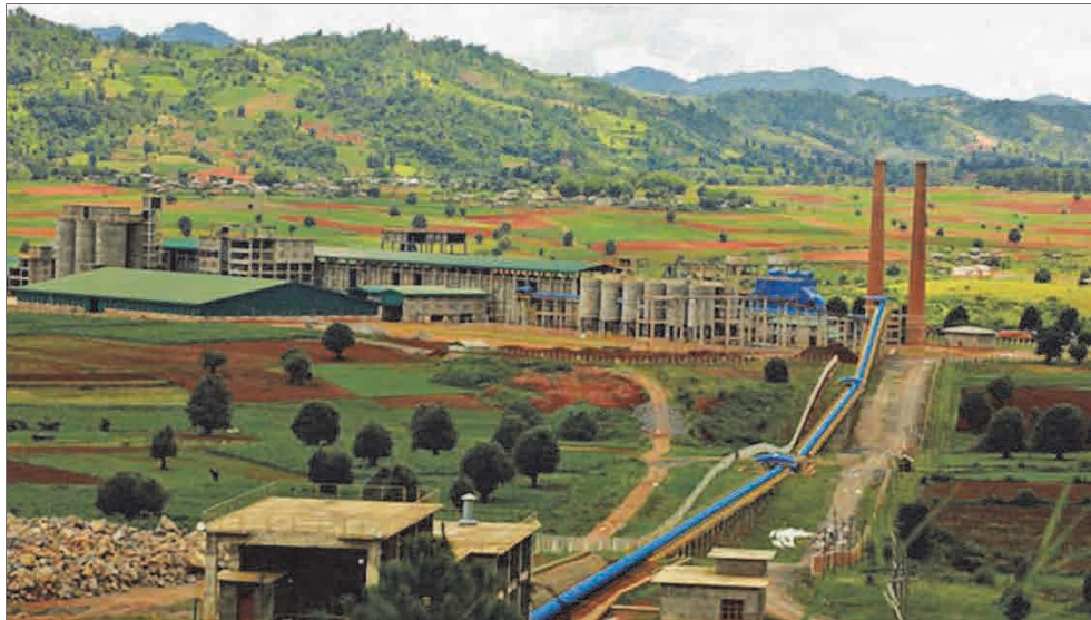
Figure 35: Dragon Cement Factory
